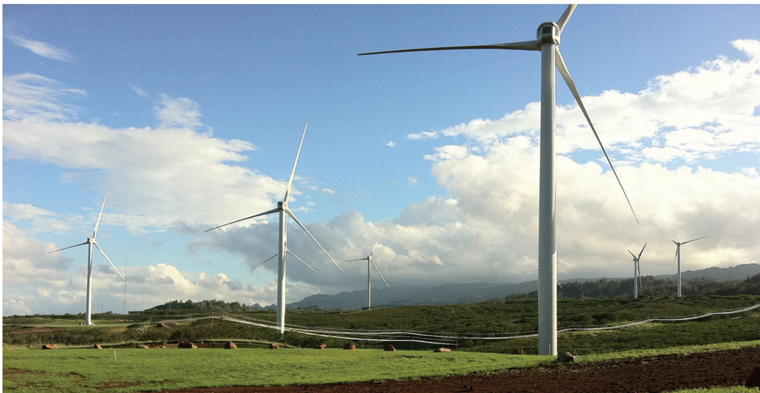
Kahuku Wind Farm in Hawaii.
