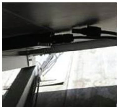
Figure 8: Failed connectors lead to loss of power production.
