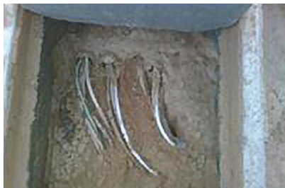
Figure 4: Dirt and water in the electrical box will trigger the inverter to shut down.
