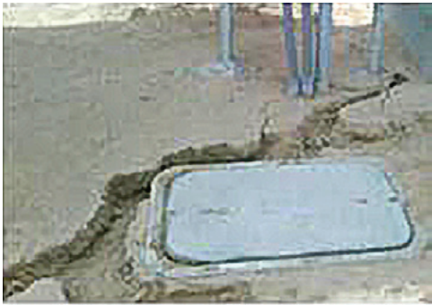
Figure 3: Heavy rain eroded the area surrounding a junction box.
