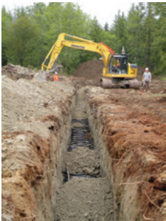
Right: Approximately 750 homes and commercial buildings will eventually be connected to a large horizontal GHX currently under construction in Gibsons, British Columbia. Homes in this climate require more heating and will extract more heat from the ground heat exchanger (GHX). Commercial buildings require more cooling and reject more heat to the GHX. Being connected to the same GHX benefits them both...it's a synergistic relationship.
