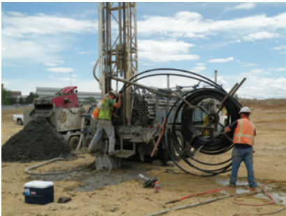
Left: GHX pipes being inserted into a borehole for the first North American IKEA Store with a GeoExchange system currently under construction in Centennial, Colorado—130 boreholes drilled to a depth of 500' will provide the heat source and cooling for the 400,000-square-foot facility.
