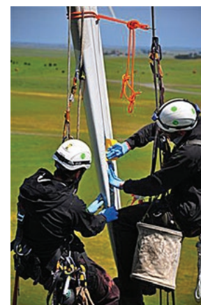
Wind turbine technicians apply wind protection tape to a blade's lead edge (Photo credit: Rope Partners; www.ropepartner.com )
