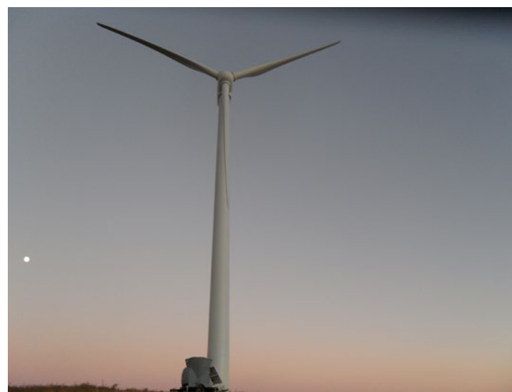
Remote sensing systems can be sited flexibly; this photo shows a Triton SoDAR at Windland's Tehachapi wind farm
