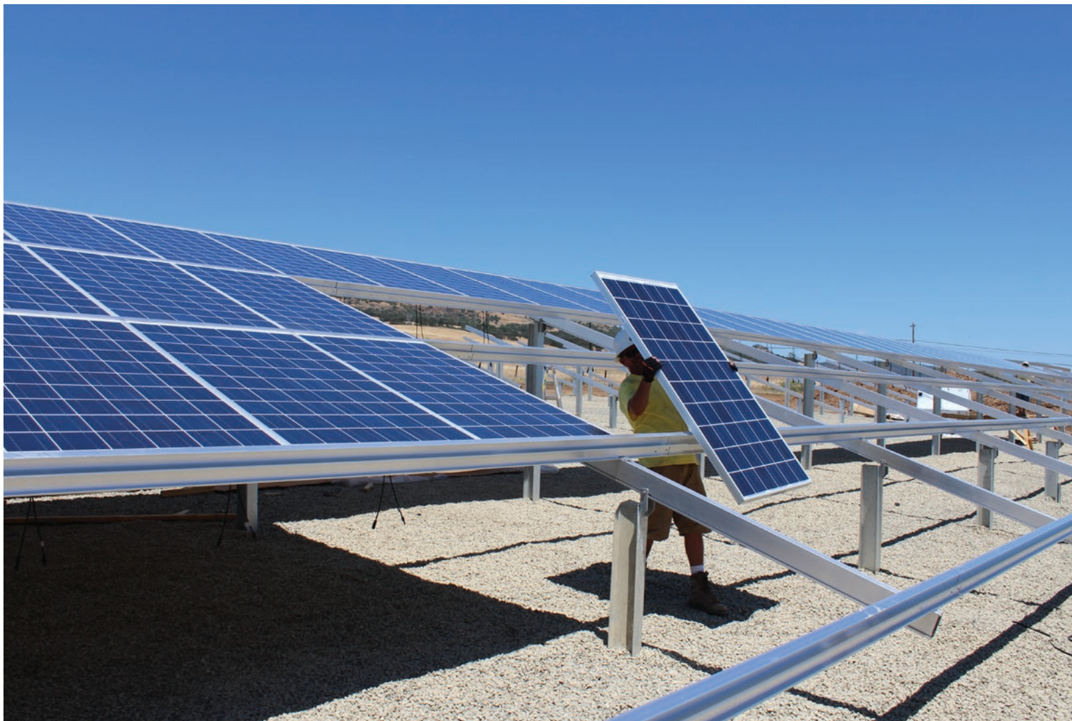
Left: Panels can be inserted from underneath the array Below: Insertion rail profile of a clampless mounting system
