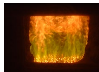
Image 4. As the volatile gasses are released from the fuel inside a furnace, they meet streams of high-pressurized air from the over-fire jets...this turbulent mixing of air and gasses completes the combustion process, releasing heat that's to be transferred within the boiler
