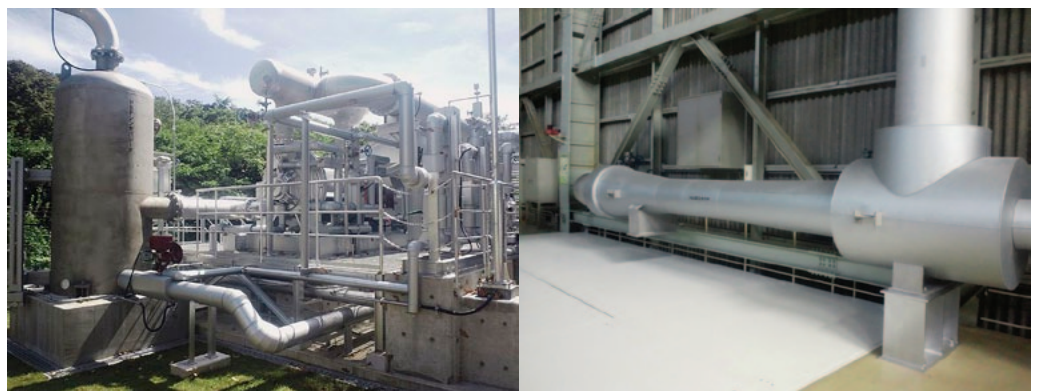
Pump 1 of the pump/ejector hybrid system
