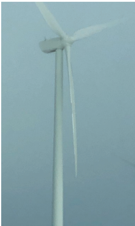
Image shows missing piece of ice from turbine blade
