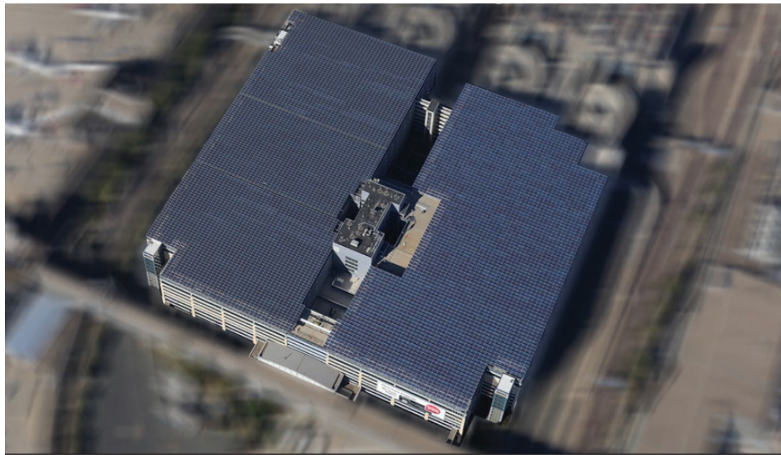
Minneapolis/St. Paul International Airport. Largest solar covered parking ramp in North America - 3.3 Mega Watts
