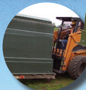
35kV 600Amp Sectionalizing Cabinets
