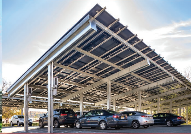
Single Post Back-to-Back SSS [Pre-Galvanized]
