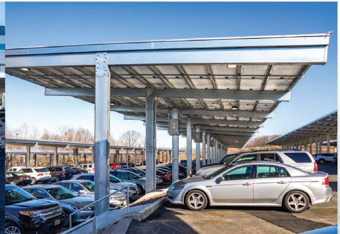
Full Cantilever T SSS Bolted Connections [Pre-Galvanized]
