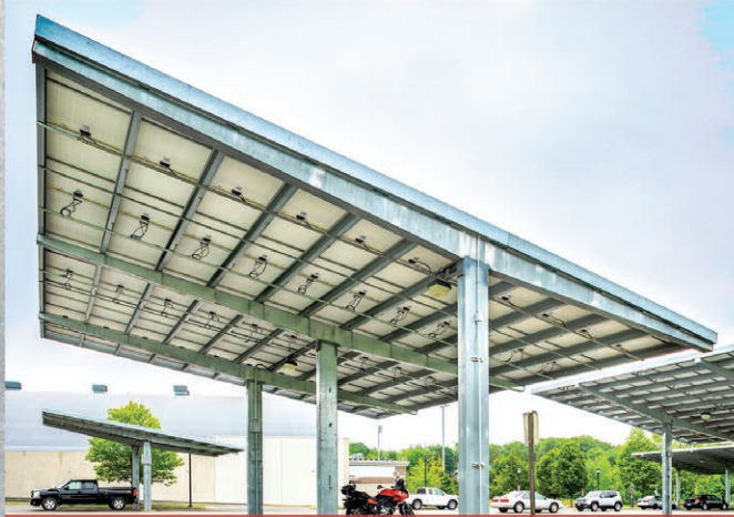
Full Cantilever T Tapered SSS [Pre-Galvanized]
