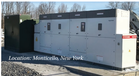
Image 7: PV inverters in cold climate
