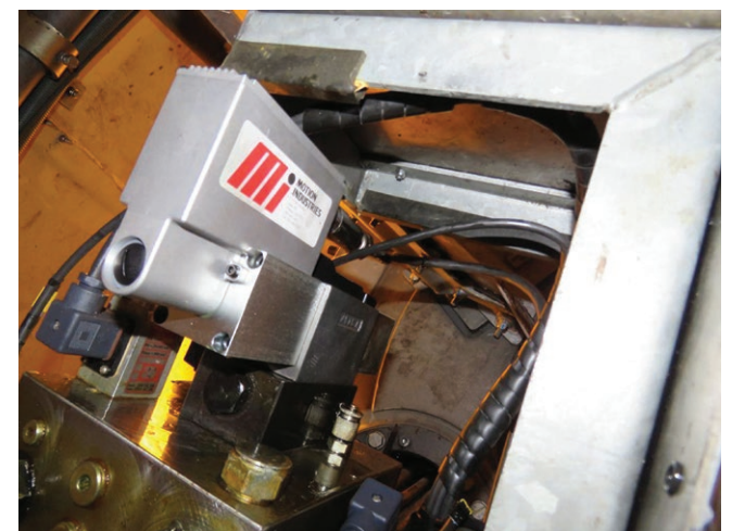
This 50-liter pitch valve was designed with a more robust electronic package to decrease failure rates in harsh operating environments.
