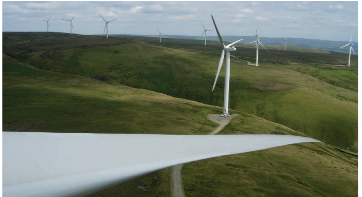
Figure 1. Yaw error can significantly impair WTG production; in the above example, a 15° yaw error resulted in a 7% loss in WTG production.
