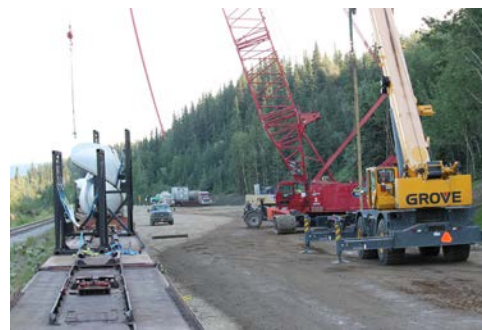
Far left: Just before midnight, a blade is attached to a wind turbine at the Eva Creek Wind Farm in Ferry, Alaska. During the height of summer, it was light nearly 24 hours a day.
