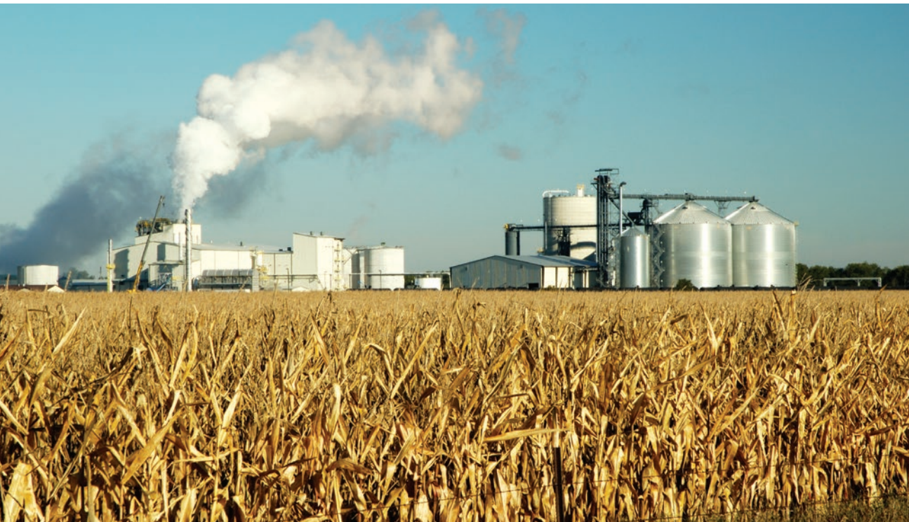
At its plant in Richardton, North Dakota, Red Trail Energy produces ethanol from corn using a dry-milling process.
