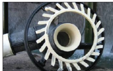
Sulfur fouling on and in the spray nozzles results in uneven water distribution over the fill.
