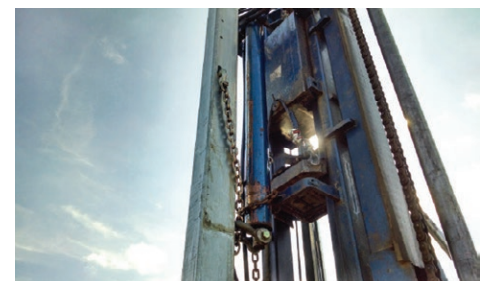
One Stop Solution for Geotech, Pull test & Turnkey Services
