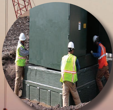
Chuted Box Pads for Pad-Mount Transformers
