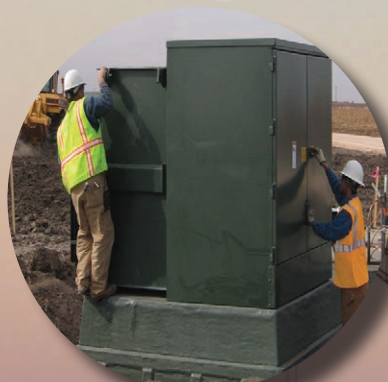
Chuted & Un-chuted Box Pads for Pad-Mount Switchgear
