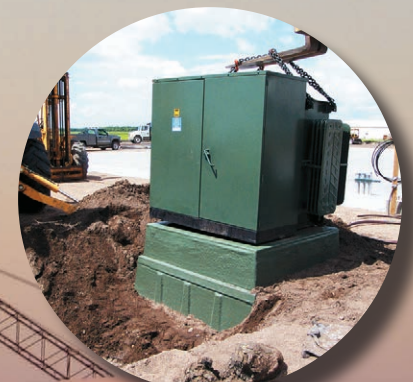
Box Pads for Pad-Mount Grounding Transformers
