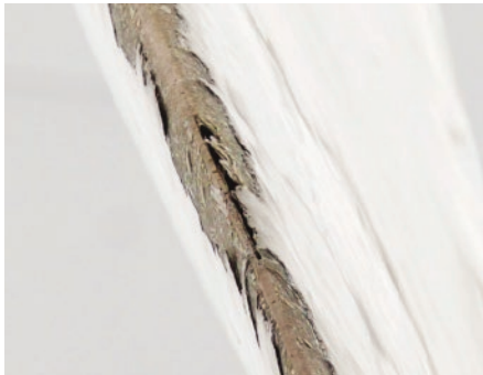
An effective blade maintenance will avert advanced stage blade erosion, impacting production and requiring extensive, costly repair.
