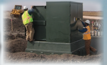
Chuted Box Pads for Pad-Mount Transformers
