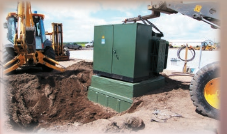
Box Pads for Pad-Mount Grounding Transformers
