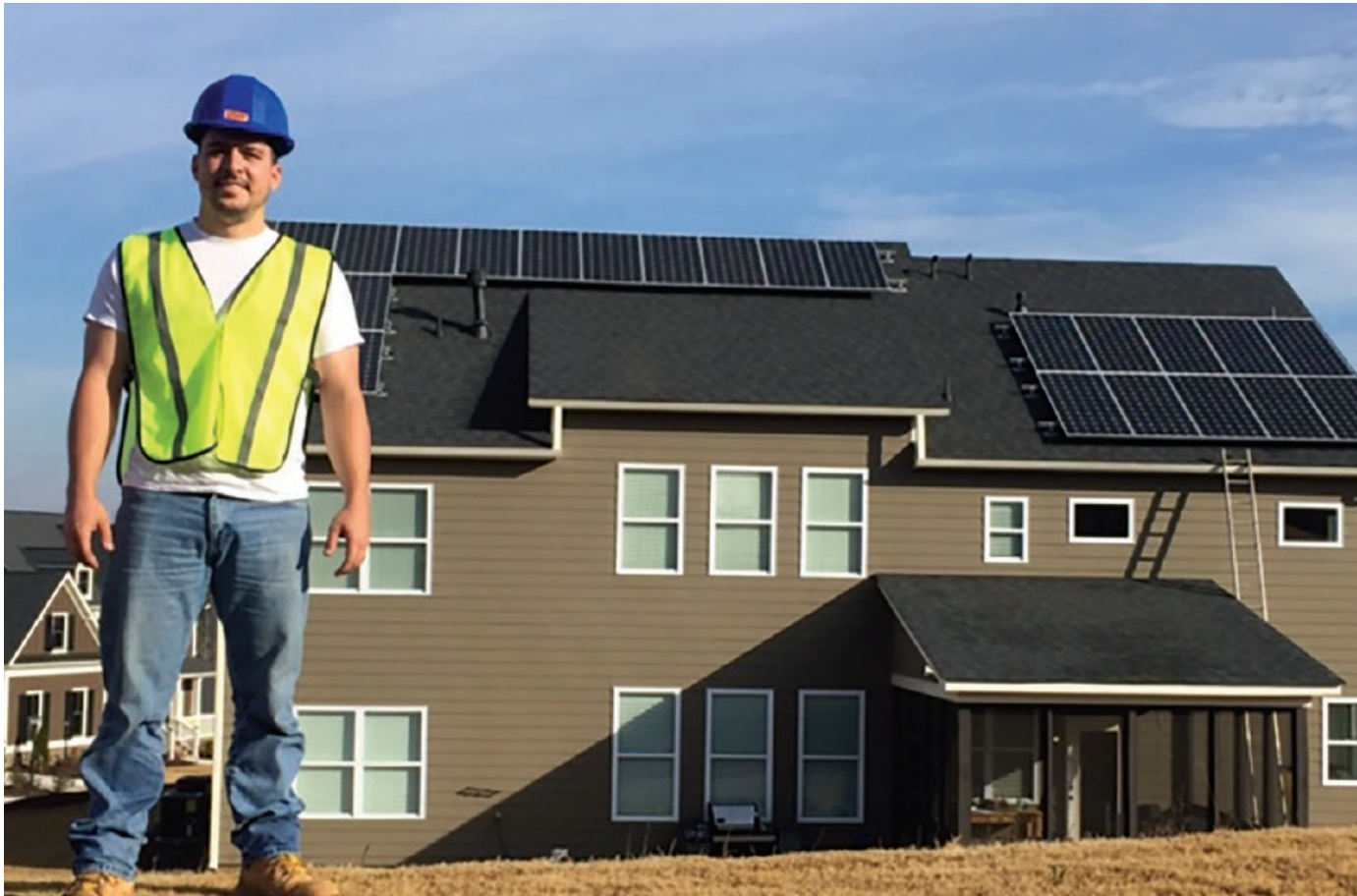
Completed residential Net Zero project. The solar installation will provide power to the home, with enough left over to charge an electric car.
