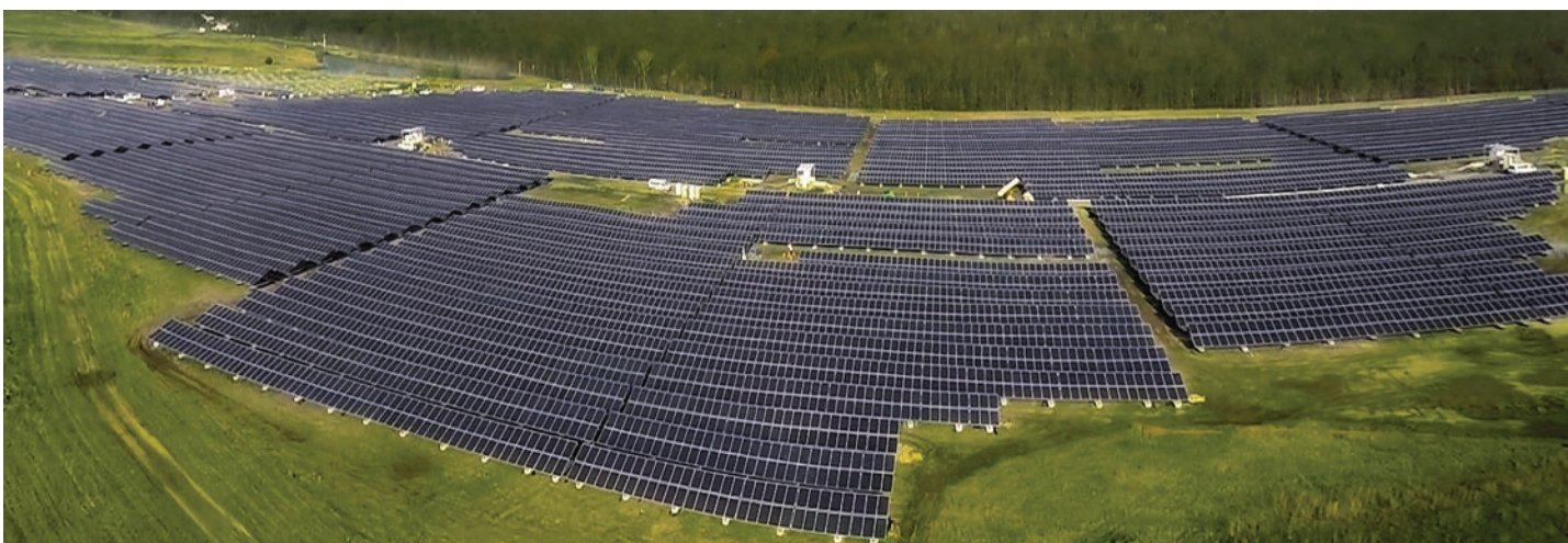
12.9 MW - NJ - Pour-in-Place™ Ballasted Ground - Largest Superfund Landfill Solar System in USA
