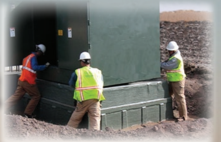
Chuted & Un-chuted Box Pads for Pad-Mount Switchgear
