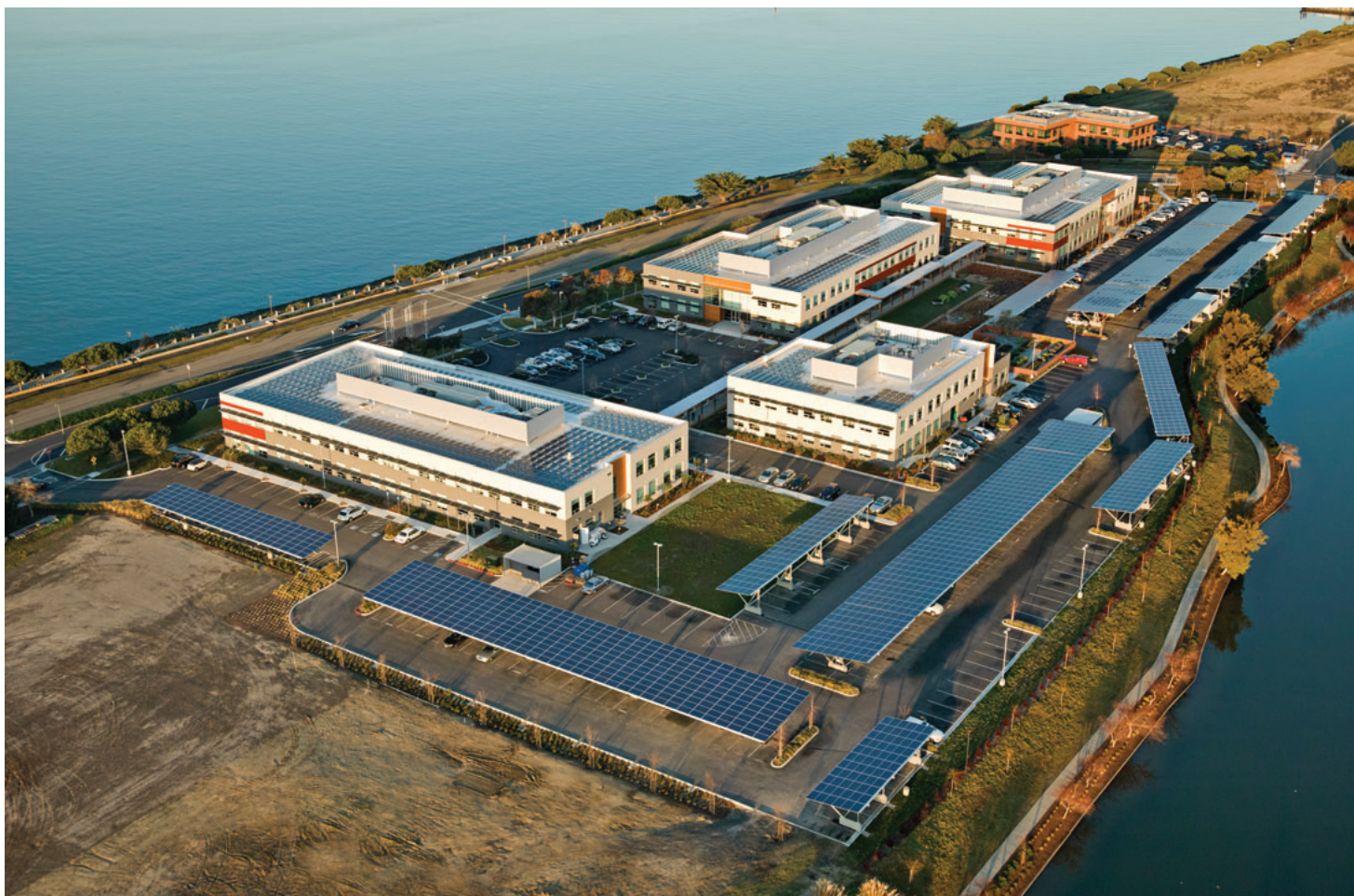
Left: VF Coalition Outdoor Campus PV project took 160 days to complete, using 39 AE 3TL three-phase string inverters (Courtesy of Hawkeye Aerial Photography)
