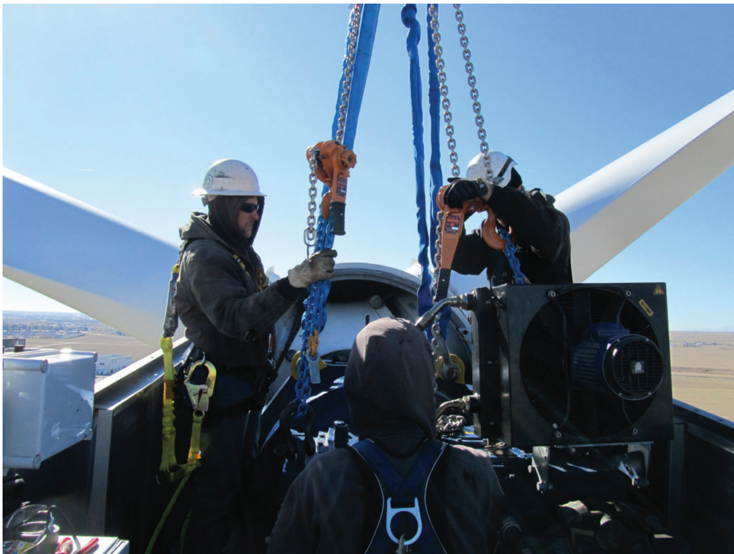
H&N Wind recently completed the build-out on this in-house rescue training platform
