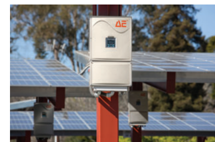
Left: VF Coalition Outdoor Campus PV project took 160 days to complete, using 39 AE 3TL three-phase string inverters (Courtesy of Hawkeye Aerial Photography)
